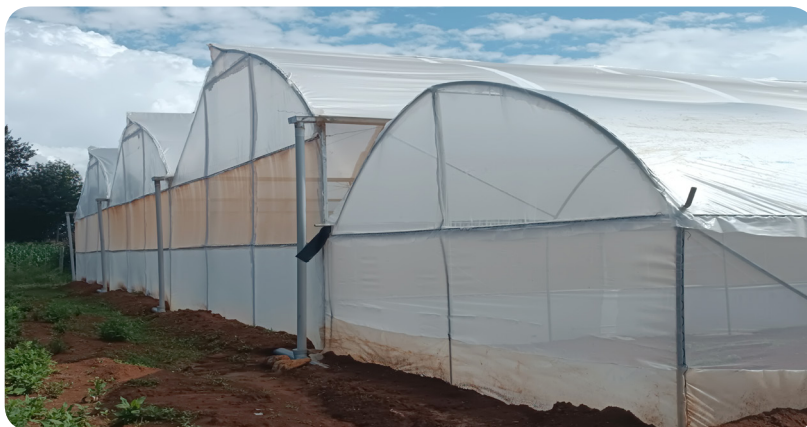
Figure 47: Galvanized steel nursery tunnel greenhouse
