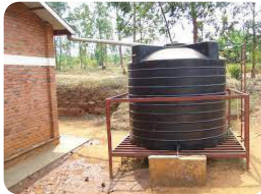
Figure 35: Roof water harvesting
