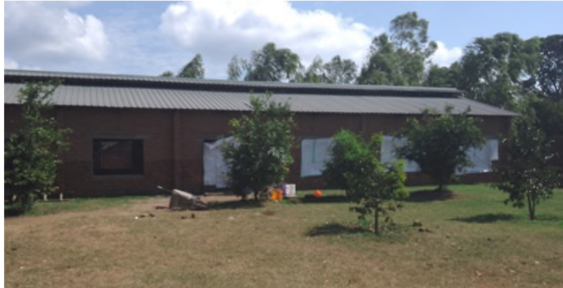
Figure 9. Broiler khola with opening at top of roof courtesy of CAPS Poultry Farm, Chinakanaka, Mulanje
