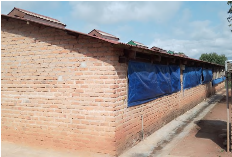
Figure 17. Brooding unit windows covered by plastic tents (tarpaulins)
