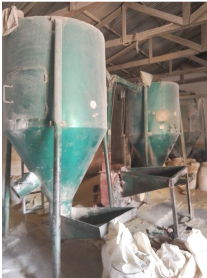
Figure 87. A purpose made feed mill with mixers, courtesy of Ndatani Premier Feeds, Lilongwe
