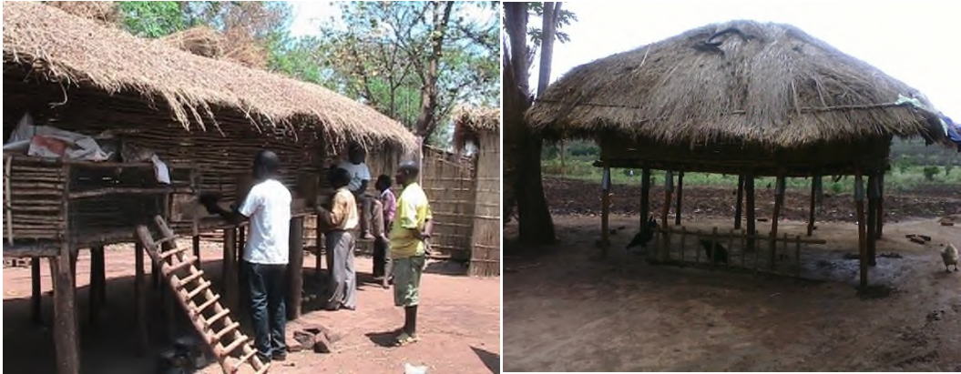
Figure 59. Left and right Elevated houses with slat floors and metal guards
